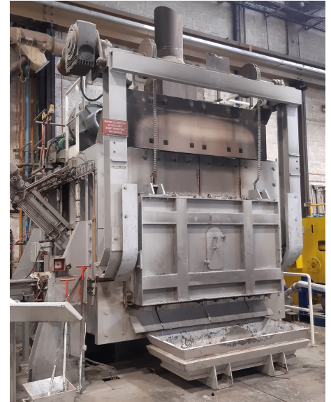
reverberatory melting furnace in use at one of Constellium's aluminum facilities.
