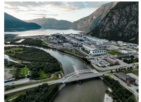
Drone photo of Sunndalsøra Norway, featuring Hydro's aluminium plant, the largest and most modern primary aluminium plant in Europe. (Photo: Hydro)
