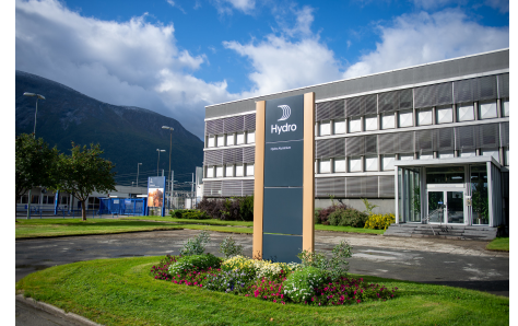
Sunndal primary aluminium plant (Photo: Anders Vindegg/Hydro)
